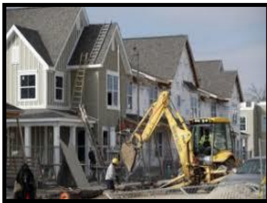
Construction on public housing development
